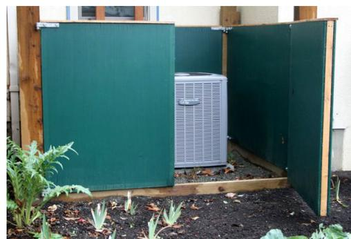
Panels are designed to fit around the heat pump or AC unit, maintaining enough space to allow servicing and maintenance. If required, Panels can be suspended on simple "L" post hinges in case they ever need to be removed. If the heat pump is in the open back yard, build the sound absorbing fence all around the pump, leaving at least 2-4 feet of space between the pump and the sound absorbing fence walls. Panels can be installed with or without cedar slats, as long as the top is
